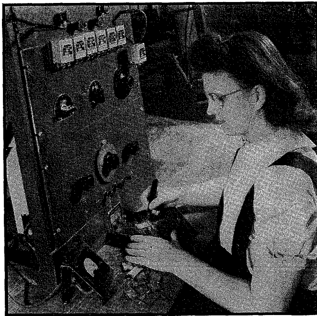
Adjusting finished silvered mica capacitors to exact capacitance value by scraping silver from the top lamination
