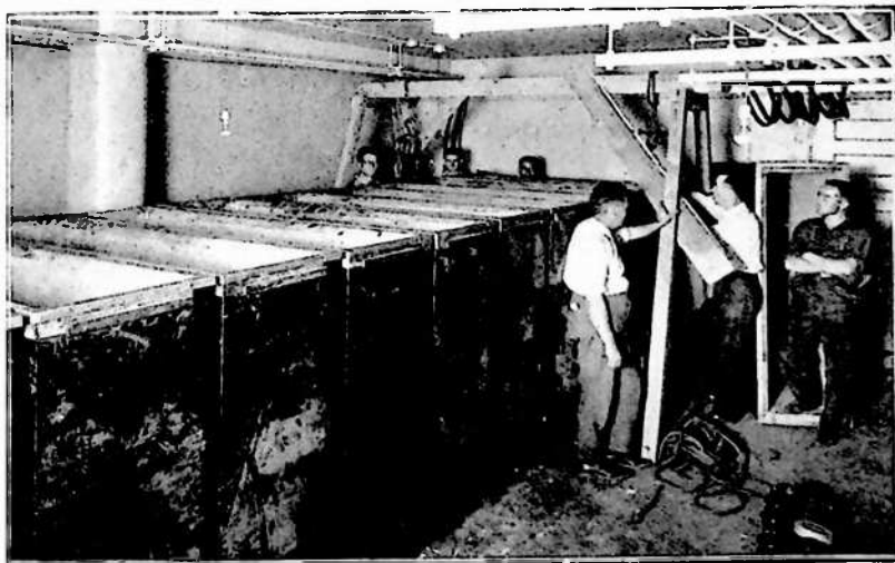
New Type H-75 Battery, consisting of eleven Cells, eleven Plates each.
