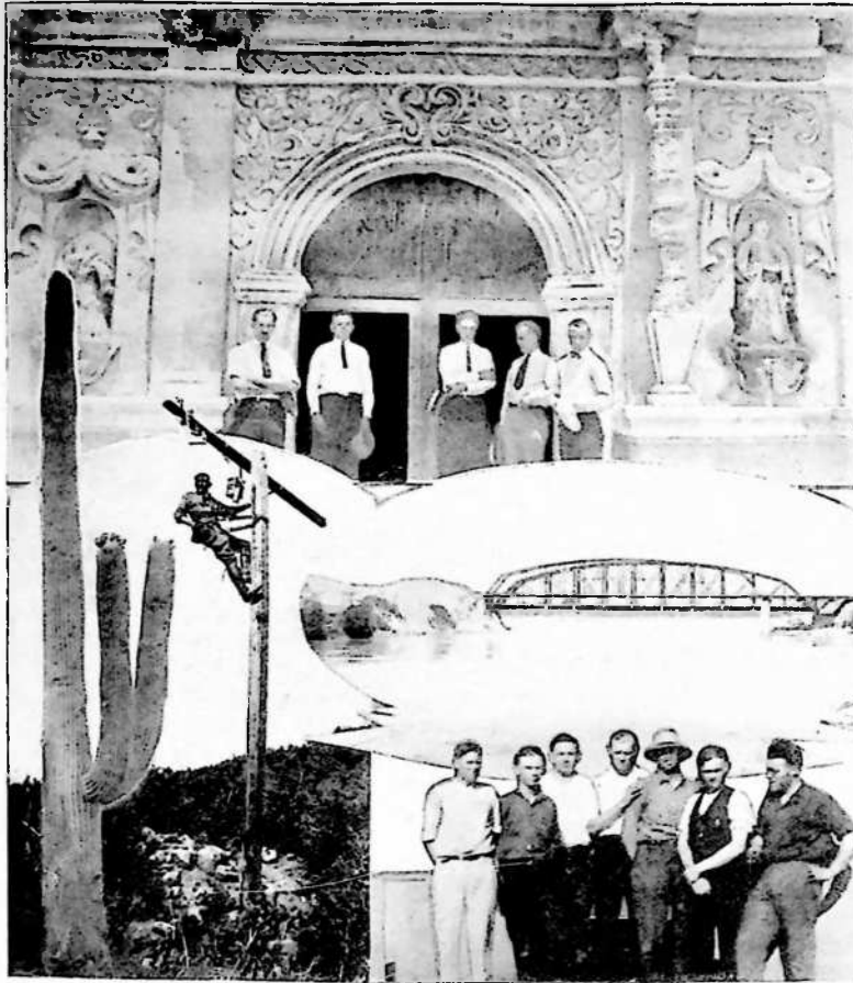
Top—Some of the Construction Gang in front of the old Mission. Lower left—Lineman up a California red cedar sawed pole 16 years old; Colorado River at Yuma, where "Foot and Mouth" victims were held up waiting fumigation. Lower, left to right—Jim Cameron, manager; Jack Robinson, local; Joe Brackett, William Verdick, installation foreman; Mr. Irwin, outside troubleman; Mr. McIntyre, toll testboard man; Don Light, power man. Lower right—Joe Brackett in flower garden beside the wall of the San Xavier Mission, Tucson, Arizona.
