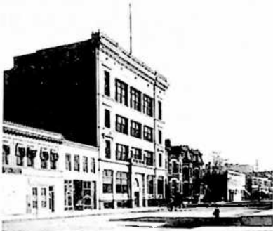
Main building in 1901, when it was but four stories high.
