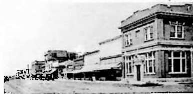
Main Street, Laurel, Montana. On right is new American Bank Building, in which the Telephone Office is located.
