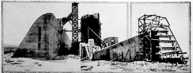
Cross-section view of the Rock Canyon dam. Right—Another view of cross-section of the dam being constructed
