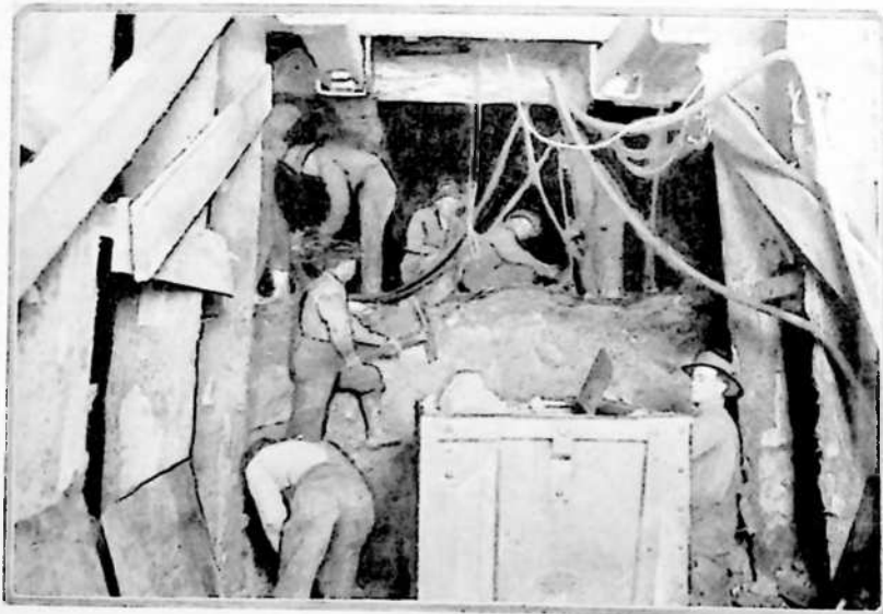
West Portal—Excavating and loading soft rock in one of the main headings
