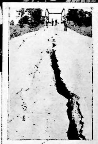
Photographs of great jagged openings torn lengthwise on the Three Forks highway, near the Jefferson River bridge, in Montana. These fissures, three and four feet wide, were many feet deep.
