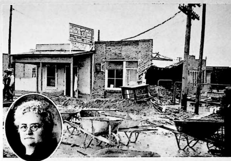
Fabens' telephone office after the walls collapsed. Mrs. Smith, operator, was faithfully at the switchboard, her clothing soaked with the flood waters, when the walls crumbled. Insert—Mrs. A. E. Smith.
