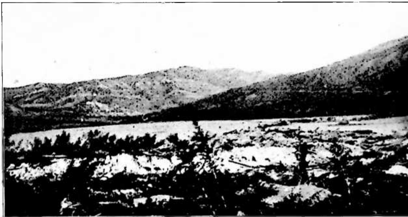
Above—General view of the great slide that filled a canyon with 300 feet of rock and dirt, and formed a lake back of it. Below—a closeup of the dam.
