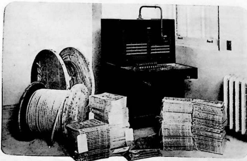
Switchboard and equipment used in the new Presbyterian Hospital, Denver
