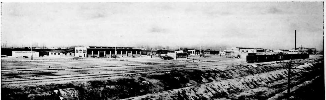
Below—Pacific Fruit Express Company's car shops recently dedicated at Nampa, Idaho. Fully equipped with telephones
