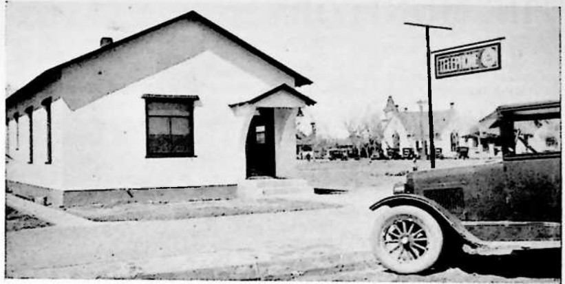
New exchange building at Ordway, Colorado
