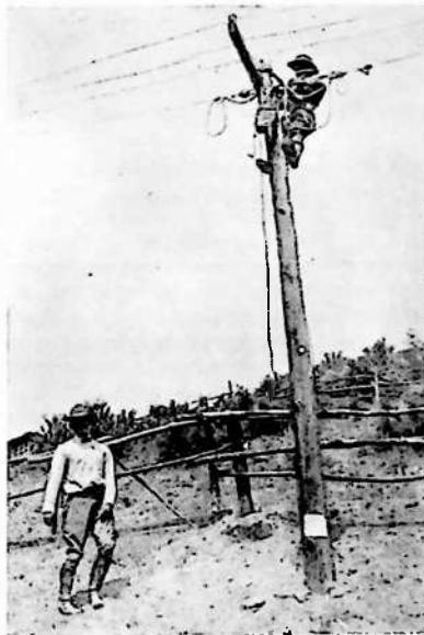
Repairing toll line trouble on Idaho City road near Morris Creek
