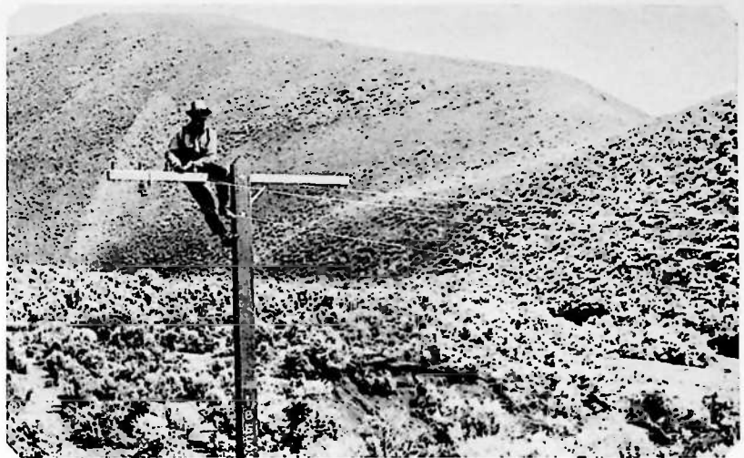
Pole 18-5-5-2 taking its place out in the sandhills to help Old Redwood carry the wires
