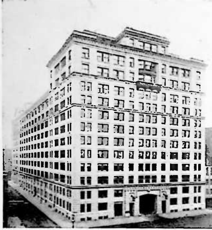
The Bell Telephone Laboratory is the sole occupant of this large building at Bethune and West Streets, New York City
