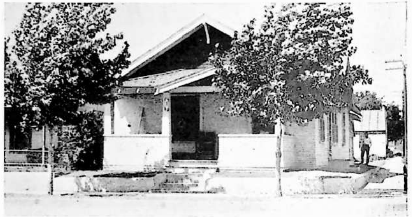
This is the new telephone exchange at Rifle, Colorado
