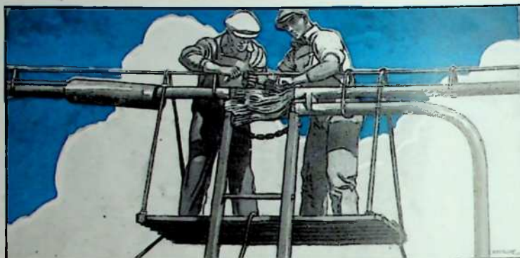
Joining the wires in a great trunk nerve between New York and Chicago
