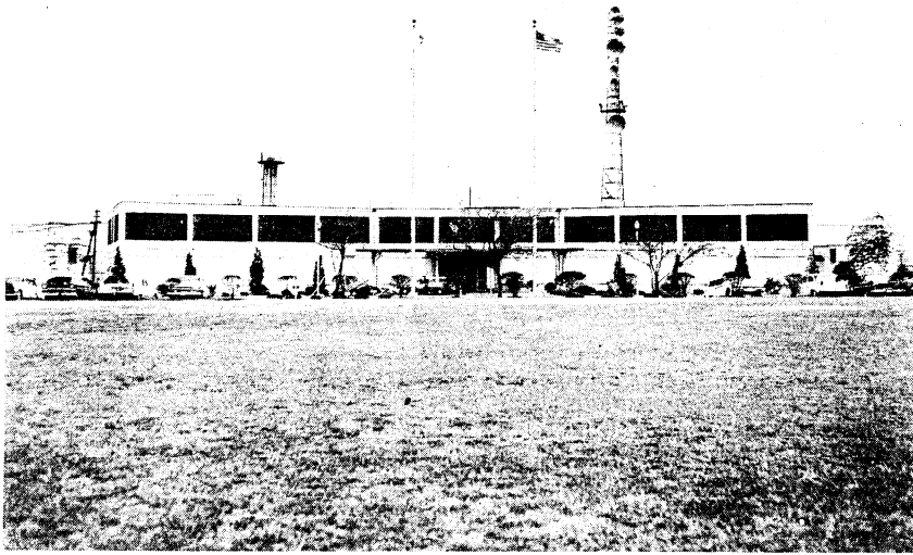
DCS Relay Station, Building 898 North Camp Drake.
