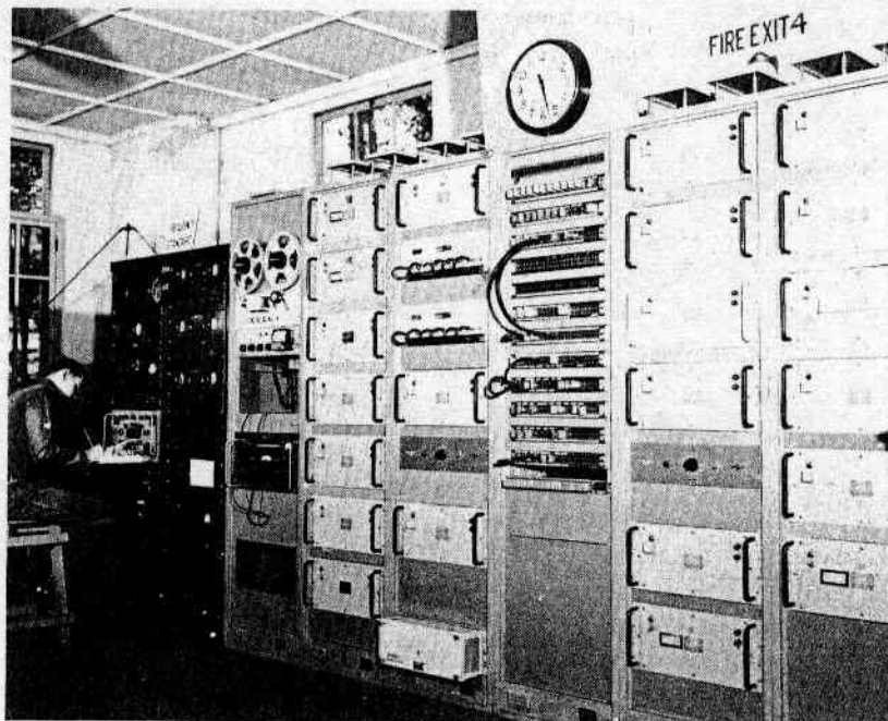
Antenna Patch Panel, Antenna Multicouplers, and Frequency Standard.
