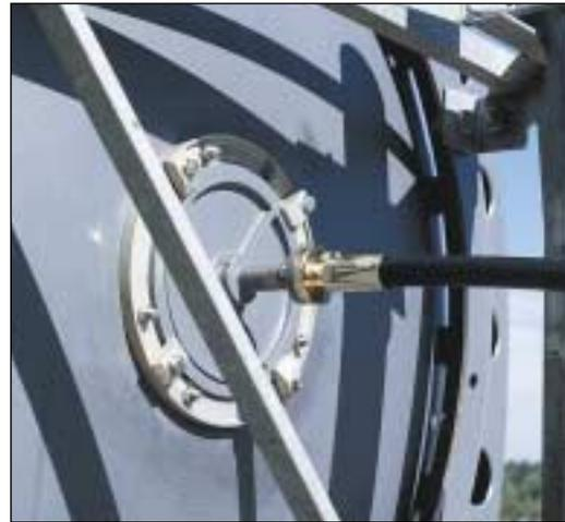
Cables and fitted connectors are available for any standard U.S., Canadian, or CCIR frequency band. Other frequency bands are available on special order. All cable assemblies are sweep tested at the factory to ensure low VSWR performance across the specified operating band.
