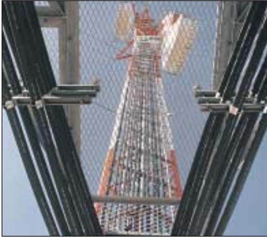
HELIAX elliptical waveguide is the optimum choice for most microwave antenna feeder systems. HELIAX is precision-formed from corrugated high-conductivity copper and has an elliptical cross section. The corrugated wall gives the waveguide excellent crush strength, light weight and good flexibility for ease of handling. A rugged black polyethylene jacket provides protection during handling and installation. A full range of waveguide sizes is available for application from 1.7 to 26.5 GHz.
