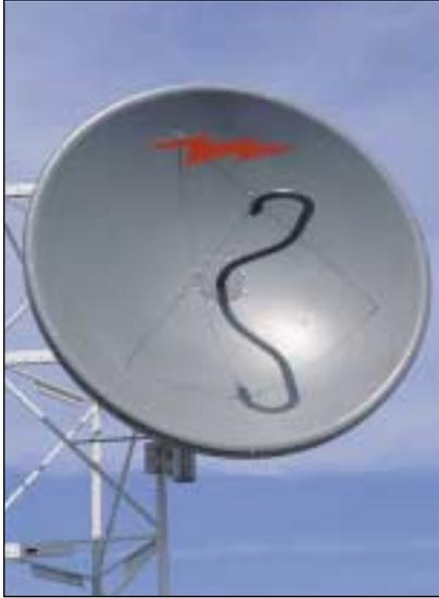
Standard Parabolic Antenna
