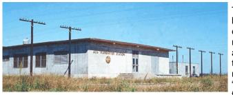
The new ADA Transmitter building is concrete, in the middle of the airfield. A 200' tower holds the microwave "dish" antennas for four 24-
