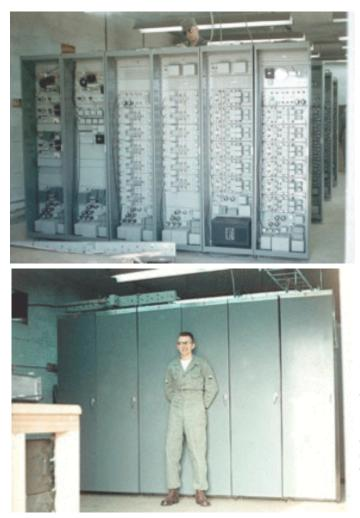
At left a wireman is installing a 24 pair telephone cable to make the 24 voice channels to the microwave patch board. This photo shows the two RF racks on the left, two transmit racks, two receive racks. Mode is pulse position modulation, 0.5 microsecond
