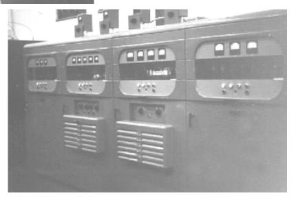
length of each wall at chest height. Final painting not completed when this photo was taken. New transmitter control console being installed, jack fields and audio
