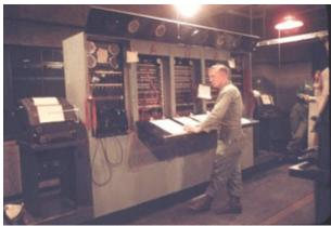
middle bank of teleprinters. Handsets for San Francisco, Honolulu, Seattle and Okinawa permit instant voice communications with them over the SSB voice channel order-wire. Behind the camera is a glass partition isolating Control from This is "Control," the Center of FEC Hq communications at Chuo Kogyo. Not a Message Center, Control oversees Transmitters, Receivers, and controls the flow of teleprinter messages to and from all the other stations in the Army's Pacific network.
