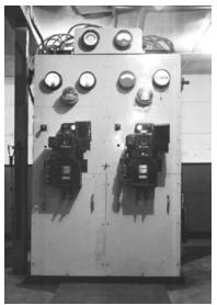
At left the main power box. Tokyo-supplied power on the left. Power demand at time of photo was 320 KW. The right side is for ADA's own emergency motorgenerators, three of the six MG sets shown
