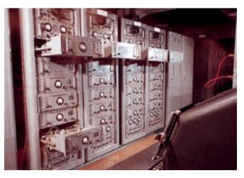
wiring were needed from time to time and such are done by moving jumper wire pairs on the "main frame" shown
