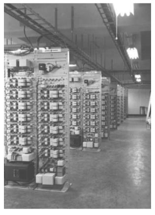
frames were crystal controlled in rate asynchronous to receive pulse frames. Channel modulation was done in the center two racks, channel modulators in pairs. Channel demodulators were also in pairs, located in the right-most racks. The frame rate allowed 3 KHz wide audio channels with each channel demod having a low-pass filter that removed any higher frequencies. Signal to noise ratio for each channel was better than 45 db.
