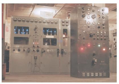
supply than transmitter. The power supply took up the left two-thirds, blue glow of mercury vapor rectifier tubes visible through windows. The final amplifier was to the right using air-cooled triodes (filament glow of one seen through the window on the right). The PW-15s were designed for commercial service before WW2. PW-15s at
