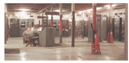
Inside the main building at the "top" of the T-shaped plan. HF Transmitters from 1 KW output to 15 KW output run along all walls. At the time of this photo there were about 36 transmitters installed.
