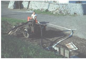
The Transmitters island of Tsukushima was very nearly at sea level. This caused seepage of sea water close to the island surface. At left SFC Joe Takahashi is operating a pump mounted on a trailer to remove water in a rock-filled capture sump around the inner perimeter ramp. Joe is the emergency power NCO and a likeable guy.
