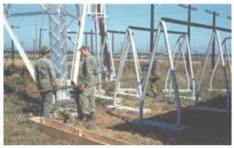
At left, Outside Plant Telephone men preparing the 20-foot rigid coax sections for the microwave feedlines. The coax is 1 5/8" diameter rigid line that will be pressurized with dried air. At right the three are up on the tower attaching the sections. The
