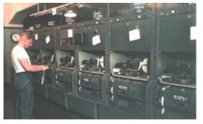
outgoing messages so they can be re-sent immediately. All outgoing tape dumps into waste bins at the bottom of each TTY rack. In the foreground is a rack of some tapes ready to resend.
