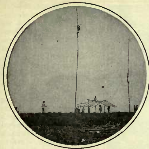
ERECTING WJS'S MASTS
