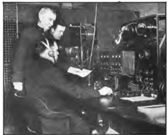
© Kadel & Herbert New York's Police Department Radio System. This installation has been of great use in calling out the reserves, when needed, and relaying messages to the police boats in the running down of bootleggers smuggling liquor. It will shortly serve to keep Police Headquarters in touch with the Department's patrol automobiles
