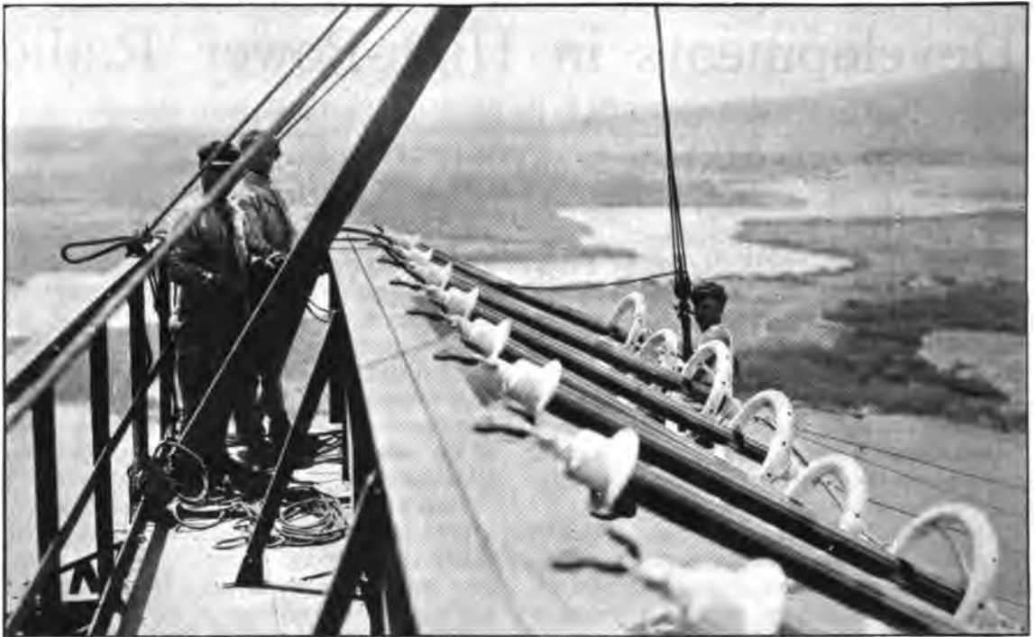
Riggers replacing a defective insulator in the Navy's Pearl Harbor high power radio station antenna
