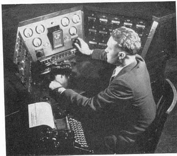
Fig. 12—Operator's control console.
