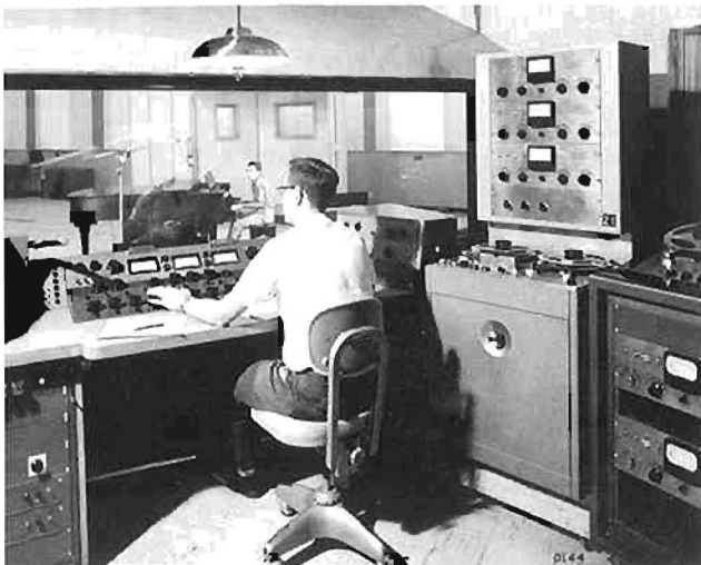
Magnetic equipment in the recording industry. Ampex Model 300-3 installed at United Recording Studios, Hollywood.
